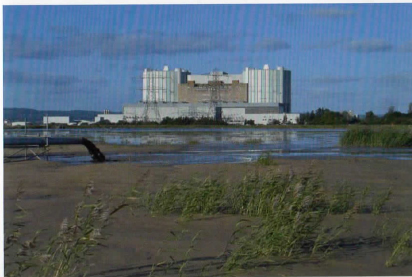
Plate 8. Lagoon 3, Oldbury Power Station.
